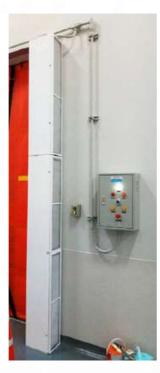
The EVA-5E-V/EVA-5SE-V series are special versions of the vertical Air Curtains series. They are designed to incorporate up to 2 filter panels.
